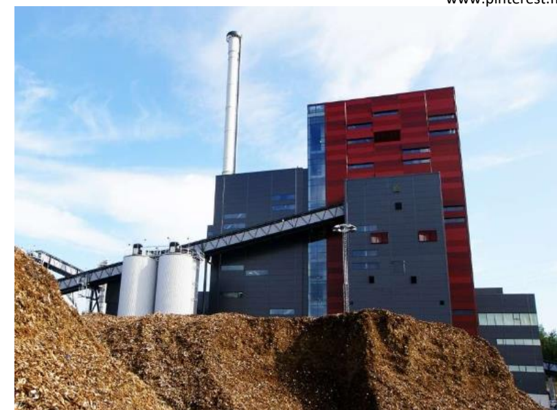
CHAUFFERIE BIOMASSE – PHOTO SUNVALOR
